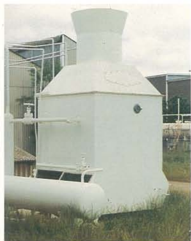
II. ENVELON applied to protect steel in aggressive chemical environment
