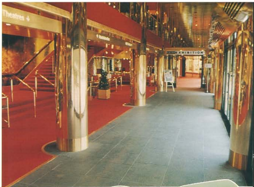
VII. Highly polished copper retains its shine and is protected against corrosion with a clear ENVELON film
